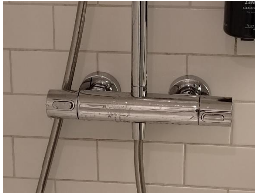
Figure 1. Shower mixer with interface elements subject to assessment using the IEC method.
